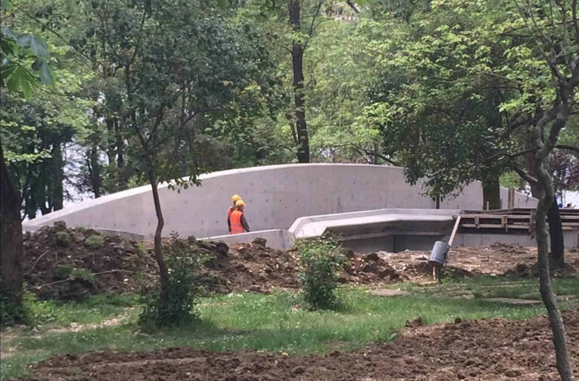
A wall filled with concrete raised inside the park.
